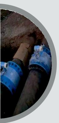
The flux density of the electromagnetic field in a given Flowmeter and the distance between the electrodes are constant. Therefore, the induced voltage is only a function of liquid velocity.
